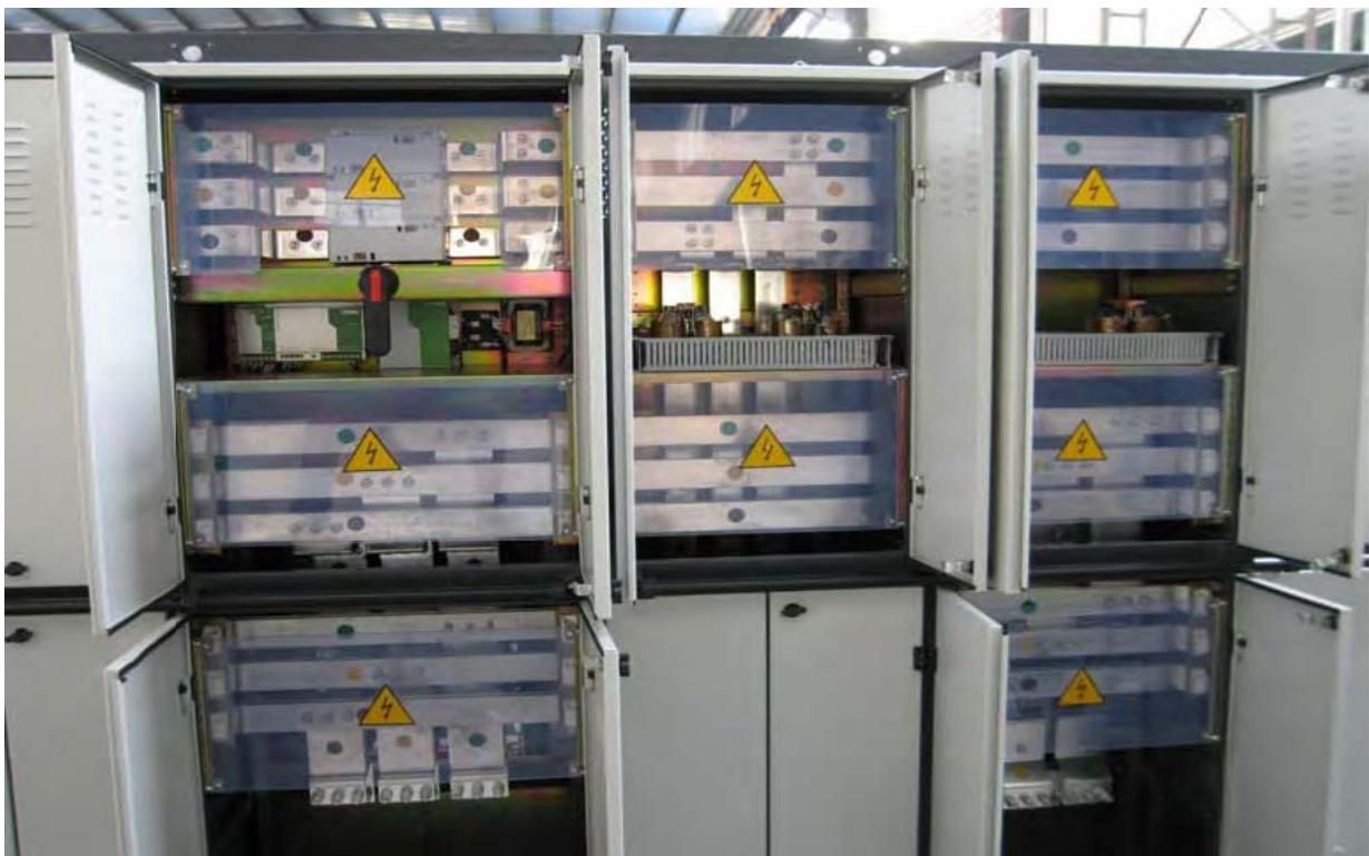
The phase mark of AC system is R-Y-B (or U-V-W, L1-L2-L3), the bus bar is respectively distinguished with green-yellow-brown labels. The polarity identification of DC system is P-N, the bus bar is distinguished with red-blue labels. Earthing bar is marked with yellow/green label. The bus bar phase R-Y-B and polarity P-N is arranged from left to right, top to below and front to rear.
